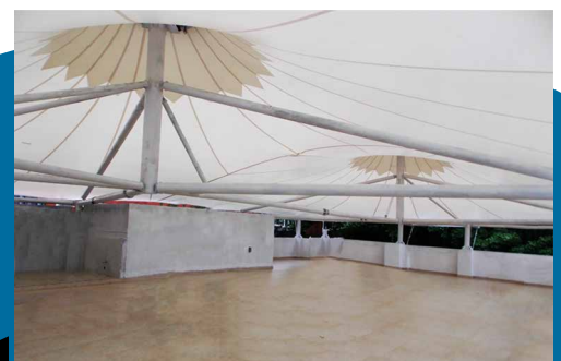
▶ Double cone center structure
