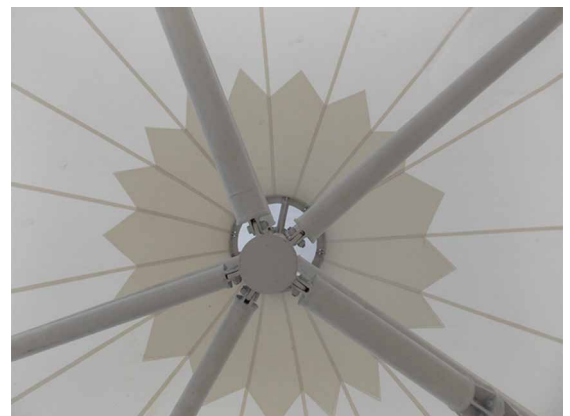
▶ Double cone center structure
